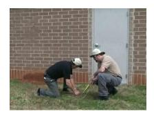
Measure and establish the boundaries of the slab using a measuring tape, spikes and string.
