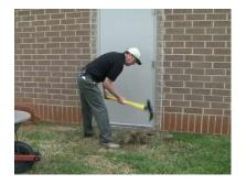
Excavate the area to remove grass and debris. Ensure that the excavated area is pitched in the direction water should run, away from any building.
