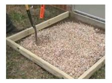
Lay a gravel base (1 to 2 inches in depth) using Sakrete All Purpose Gravel. This will help with any water flow or substrate movement and prevent the concrete from buckling.
