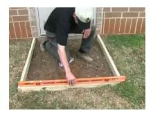
Add forms using 2x4s and ensure they are level. Nail the forms together and remove the string.
