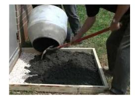
Pour concrete mixture into forms and begin spreading.
