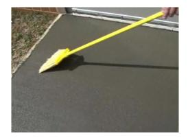
Using an ordinary broom, lay it on the surface of the slab and gently drag it across the surface to create a textured, non-skid finish.
