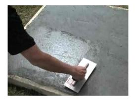
Once the wet sheen of the concrete has disappeared, apply the final trowel coat.
