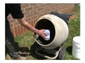
Add water as needed, 3.5 to 4 quarts of water depending on the type of concrete mix. Concrete can be mixed in a wheelbarrow, mortar pan or a mixer. Add enough water so mixture moves freely and does not ball up.
