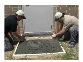
Use a 2x4 to screed the surface with a rocking motion eliminating any voids and removing excess product.
